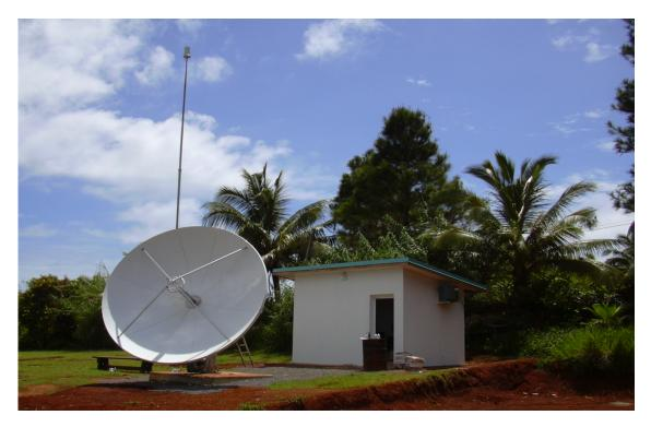
The satellite earth station with outdoor shelter allows monitoring, control, billing and access rights to the network. The 30 meter mast shown above covers the whole of the island. Repeaters are placed at strategic locations to 'mesh' back to the base station. These repeaters penetrate vegetation successfully and ensure coverage is consistent.
